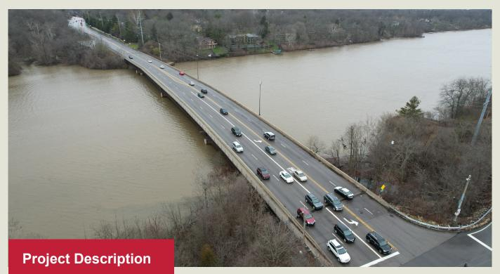
The Franklin County Engineer is rehabilitating the Hayden Run Road Bridge over the Scioto River. This project includes resurfacing of Hayden Run Road, light pole replacement, and lane width reductions to accommodate the addition of a shared-use path on the south side of the roadway.
