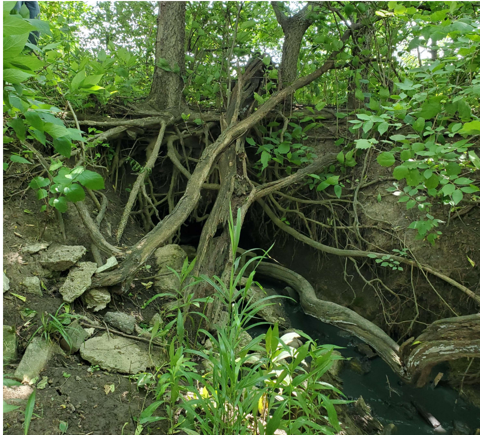
Figure 2: Severe Erosion Occurring at Outlet to Hamilton Ditch
