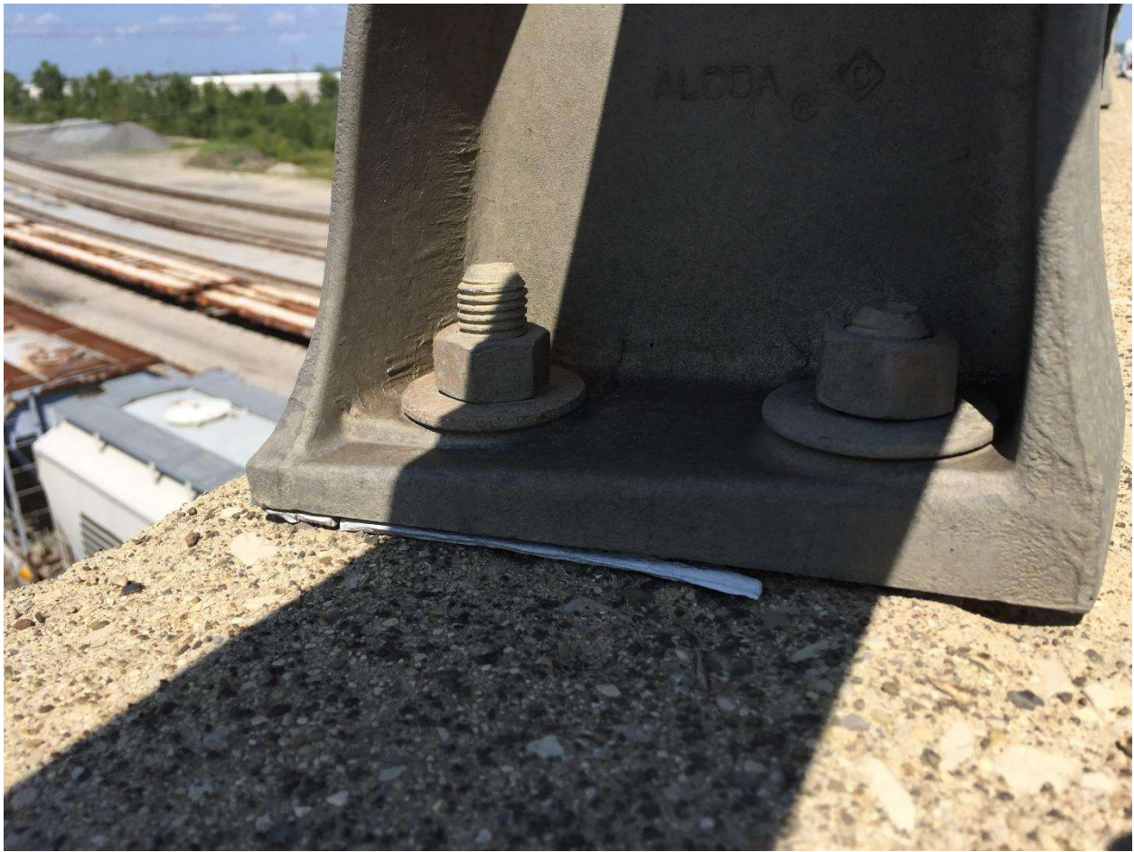
Photo #3: View of HA #3 - Non-asbestos-containing guard rail post caulking.
