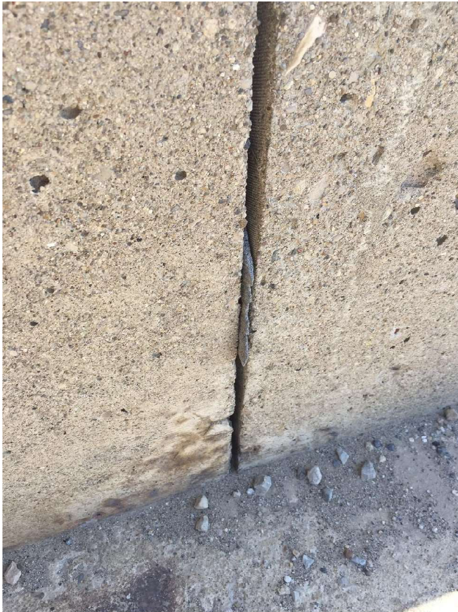
Photo #2: View of HA #2 - Non-asbestos-containing parapet wall grout.
