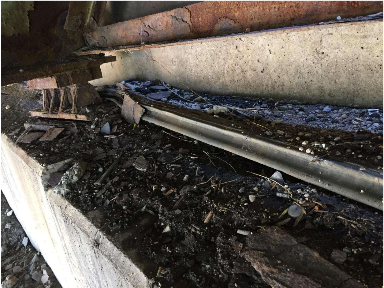
Photo #4: View of HA #4 - Non-asbestos-containing bridge expansion joint.
