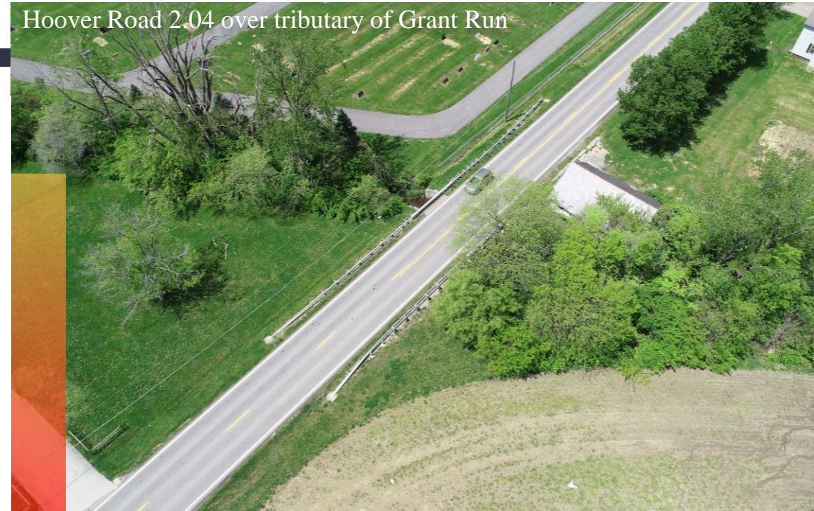
Schleppi Road 0.97 over tributary of Rocky Fork Creek
