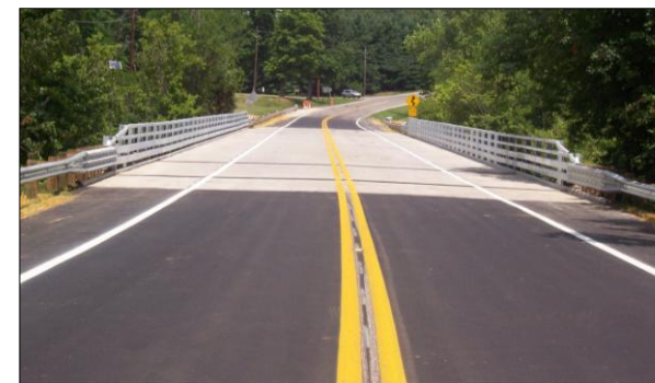
Central College Road Bridge Rehabilitation completed in July 2010
