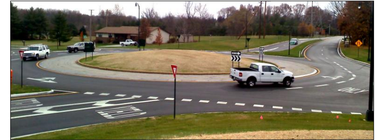
Newly built Reynoldsburg-New Albany Road and Morse Road Roundabout
