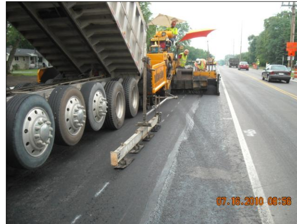
Clime Road Pavement Construction
