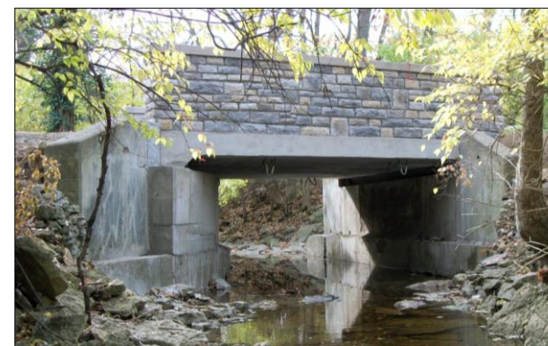
New Stoney Bridge Lane Bridge
